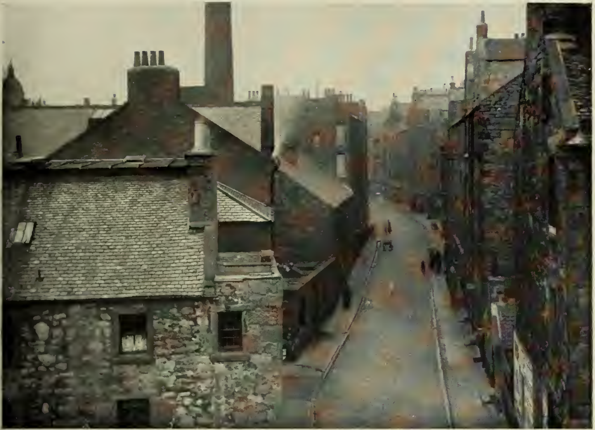
Houses scheduled for Demolition under the St. Leonard's Improvement Scheme.
